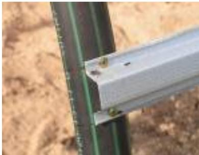
Photo 7, connect battens to arch
